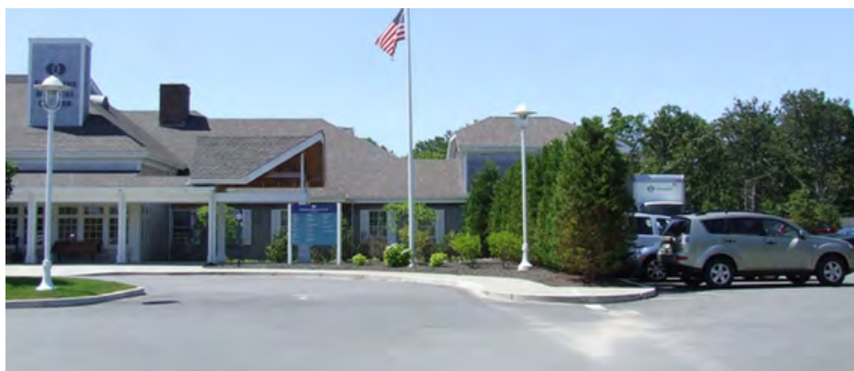
At Fontaine Medical Center in Harwich, the delivery area (right) is shielded from the public entrance to the building (left) by a narrow but dense screen of trees. Source: Cape Cod Commission
