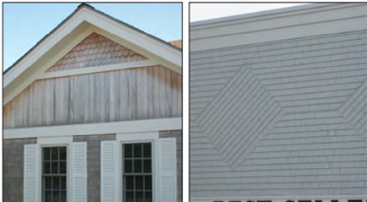
Simple changes in the pattern of the exterior materials and the use of bands of varied materials can create interest in the facades, as shown in these Harwich examples. Source: Cape Cod Commission
