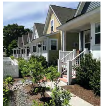
Stormwater infrastructure and native plantings integrated into the common spaces
