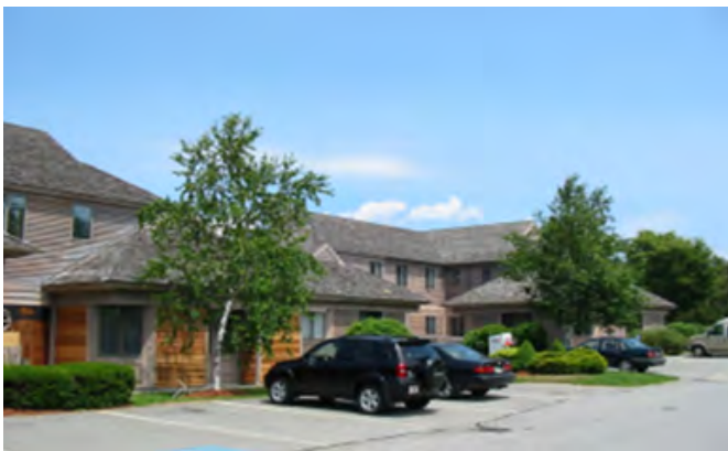
The varied wall heights on this traditional building reduces the visible bulk on a large structure. Source: Cape Cod Commission
