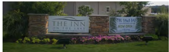
Monument sign foundational structures should be constructed of masonry materials Source: Brovitz Planning LLC
