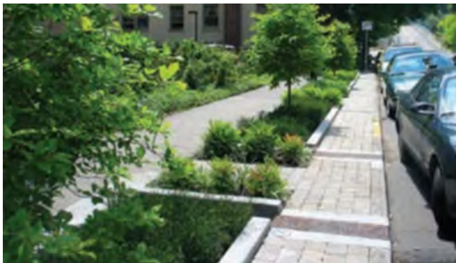
Layers of plantings through pedestrian areas also serve as stormwater management areas. Source: Vermont Urban and Community Forestry Program
