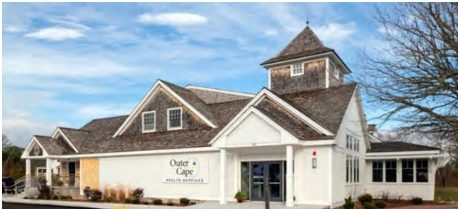
This design uses varied eave lines and ridge heights to reduce the apparent mass of the building. Source: Delphi Construction.
