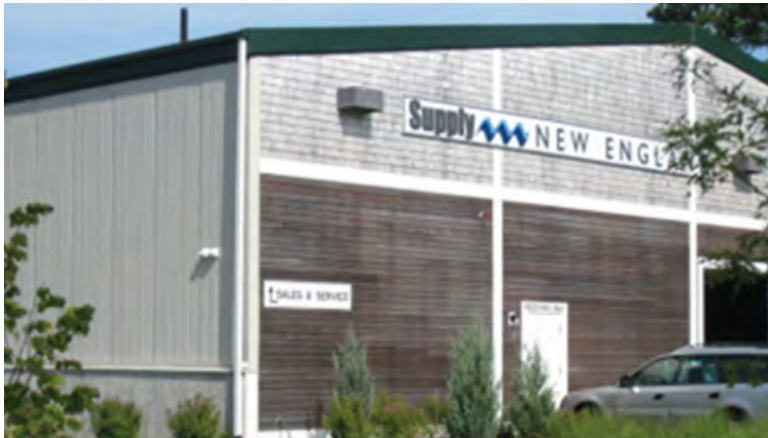
This building in Yarmouth uses a mix of traditional materials on the most visible facades and low-reflective siding in neutral tones on the side façade. Source: Cape Cod Commission
