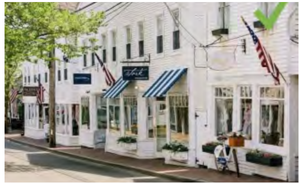
Consistent sign sizes in multi-tenant building Source: visitedgartown.org
