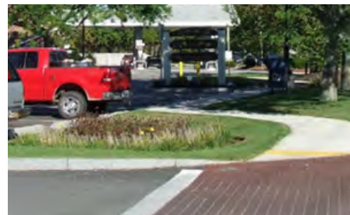
Stamped concrete enhances pedestrian safety Source: Cape Cod Commission
