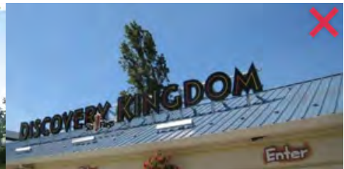
Example of wall sign that is inappropriately mounted on a track and not recommended.
