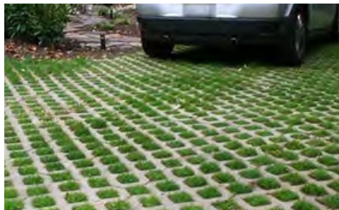
"Grasscrete" and permeable pavement allow rainwater to naturally leach into the ground and recharge the water table.
