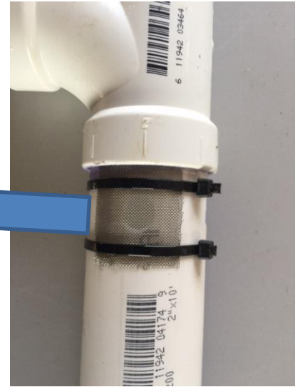
Stainless screen over relief hole
