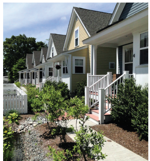
Stormwater infrastructure and native plantings integrated into the common spaces at Cottages on Greene, East Greenwich, Rhode Island.
