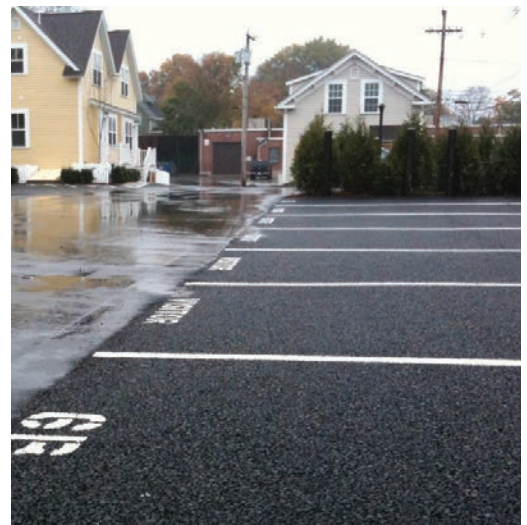
Permeable pavement used for parking spaces.
