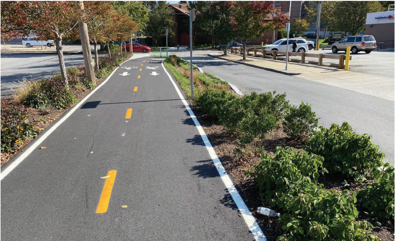
Shared use path with green stormwater infrastructure.
