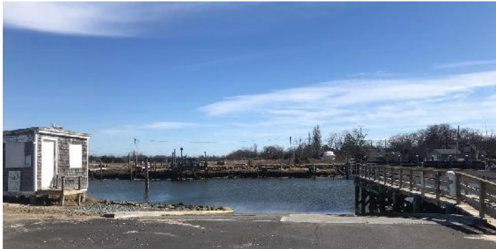
Boat launch at Rock Harbor
