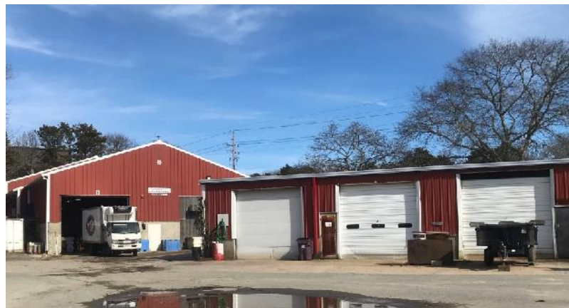
Commercial bays on Holmes Road
