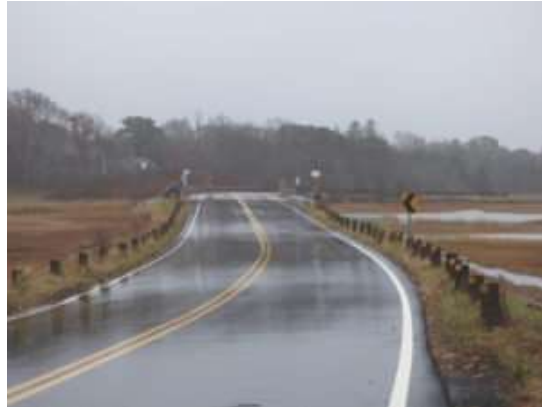
Bridge Road in Eastham is a flood
