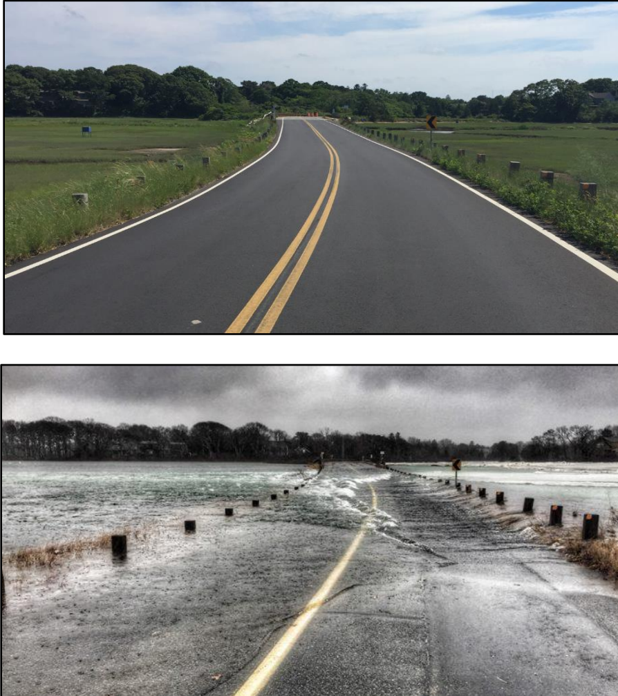
Figure 3. Calm and flood conditions along Bridge Road.
